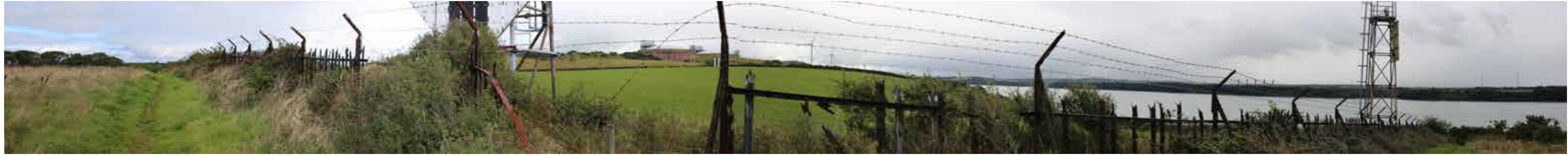
SITE CONTEXT PHOTOGRAPH 6: VIEW EAST FROM WELSH COASTAL PATH / PROW PP51/22/1 PANORAMIC PHOTOGRAPH: NOT TO SCALE AND FOR CONTEXT ONLY
